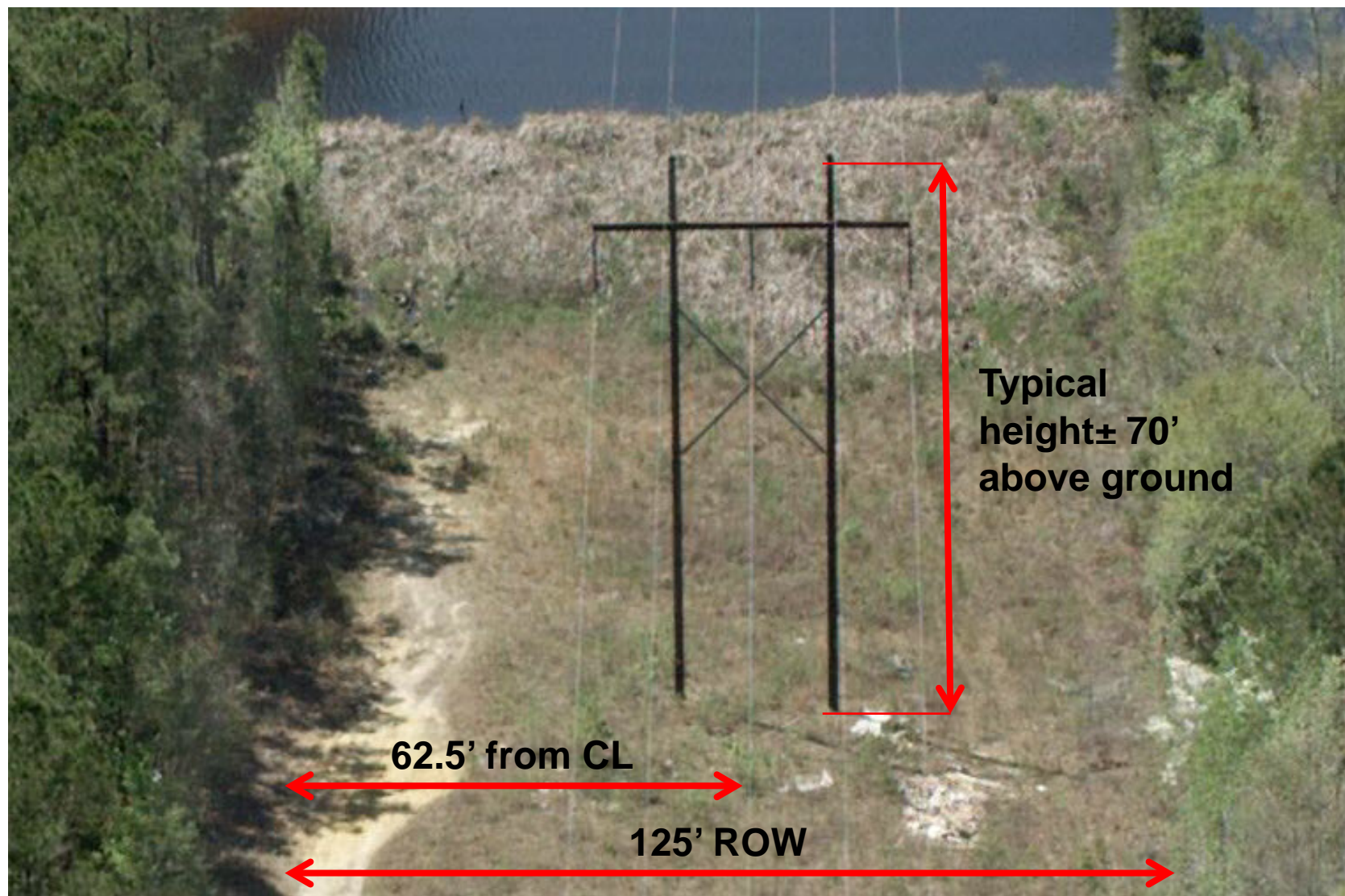
Figure 2-3: Typical Steel H-Frame Tangent Structure
