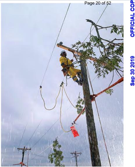
**LINEMAN IN RAIN** IN AREAS INACCESSIBLE BY BUCKET TRUCK, LINEMEN HAVE TO CLIMB POLES TO MAKE REPAIR
