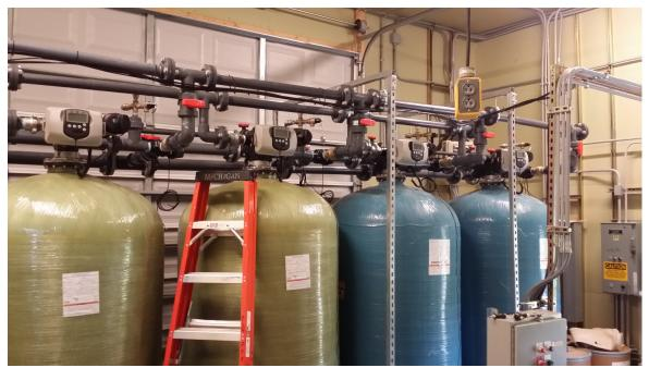
The two blue vessels and the alarm panel in front of them are part of the decommissioned uranium removal system for well 1.
