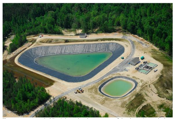
The water treatment building is located at the center top of the above picture, the long term storage pond is in the middle, the operations building to its right, and the water reclamation plant to the right of the operations building. The small square pond in the foreground is the upset pond. For scale, the small white object between the ops building and the upset pond is a full-size pick-up truck.
