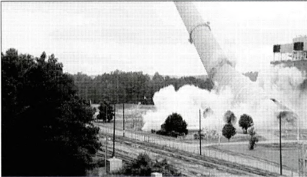
Figure A-8 Explosives Were Used to Lay the Plant Arkwright Chimney to the Ground (View 2).
