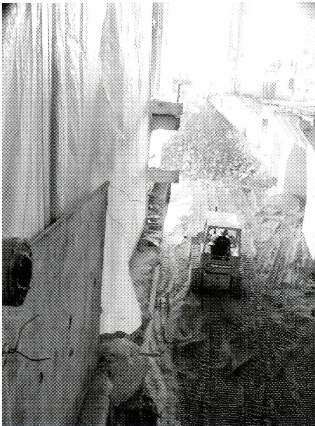
Figure A-6 Plant Arkwright During Filling of Powerhouse Basement Cavities. A ramp was constructed to fill the basement to grade level.
