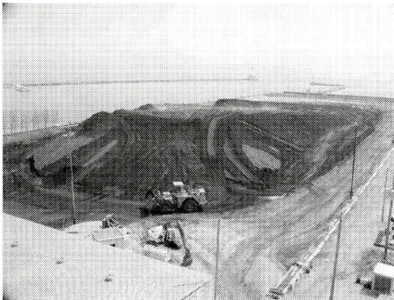
Figure C-7 Port Washington Power Plant Coal Dock. The 1000 ft long coal dock was originally constructed in 1935 from 275,000 cubic yards of dirt from a bluff on the Lake Michigan shoreline that made room for the plant.
