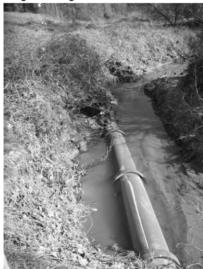
Figure 1. Exposed Pipe in Streambed
