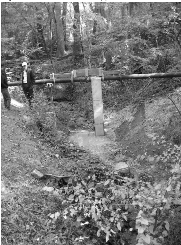
Figure 3 Bank Scour Causing Un-supported Lengths of Aerial Pipe
