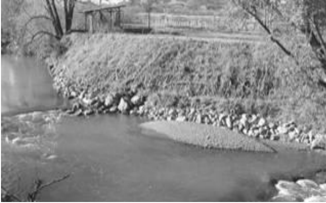
Figure 11. Streambank Using a Boulder Toe for Stabilization
