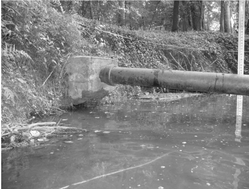
Figure 2. Scour Under a Support
