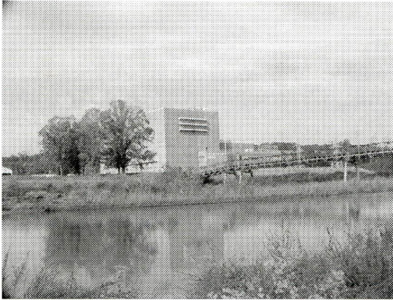
Figure B-2 Watts Bar Fossil Plant Powerhouse. Coal conveyor with Transite Panels Removed is Shown on the Right. The coal-fired plant used 82 acres of the 1067 acre site. Also on the site are a nuclear and a hydro plant.
