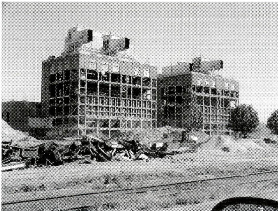
Figure A-2 Plant Arkwright During Dismantling of Powerhouses. The four 40 MW units date from 1941 to 1948. There was one stack.
