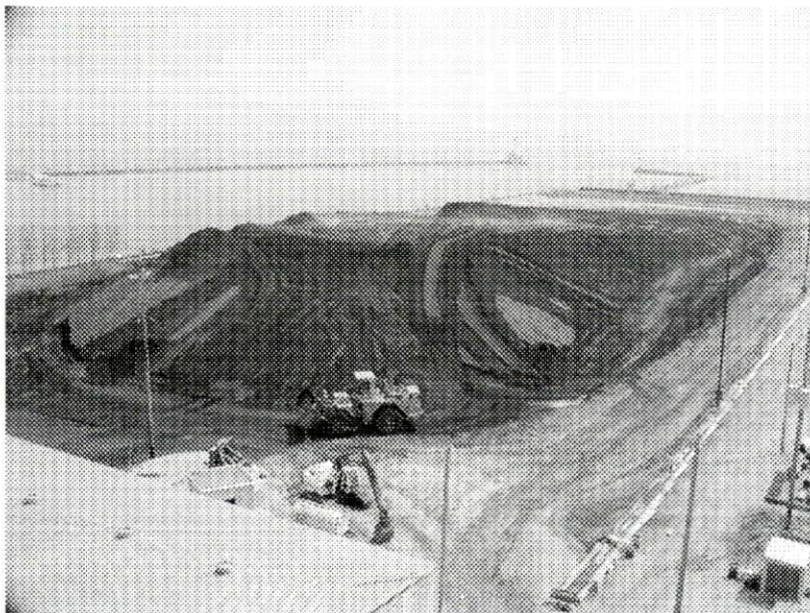
Figure C-7 Port Washington Power Plant Coal Dock. The 1000 ft long coal dock was originally constructed in 1935 from 275,000 cubic yards of dirt from a bluff on the Lake Michigan shoreline that made room for the plant.
