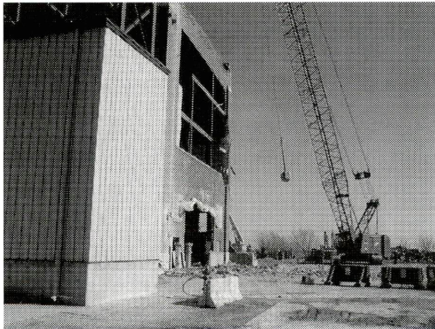
Figure C-11 Port Washington Power Plant - Demolition of Unit 5 South Wall Brick with Wrecking Ball
