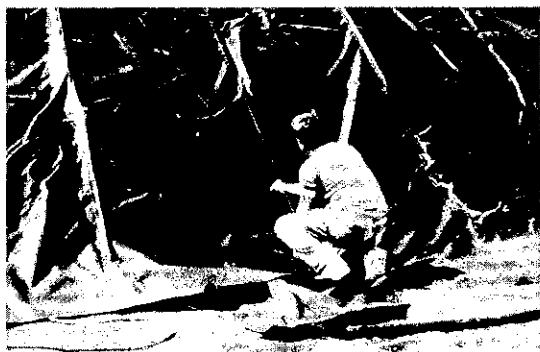
Figure A-35. Use of a chalk line to mark a liner for removal of excess material.
