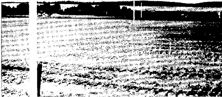
Figure A-71. Surface cover for a landfill showing gas vent pipes.
