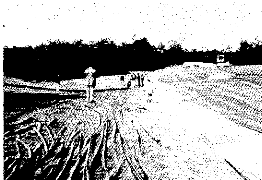
Figure A-49. Use of cover material in place of sandbags.
