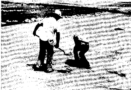
Figure A-7. Workmen removing small rocks during subgrade inspection.
