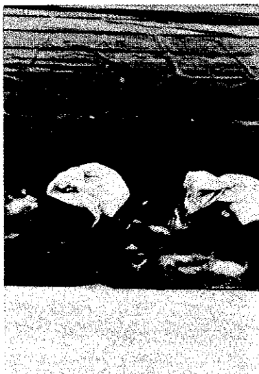
Figure A-25. Large wrinkle at edge of liner panel.
