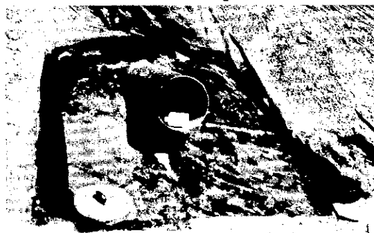
Figure A-36. Field constructed boot for a liner penetration.
