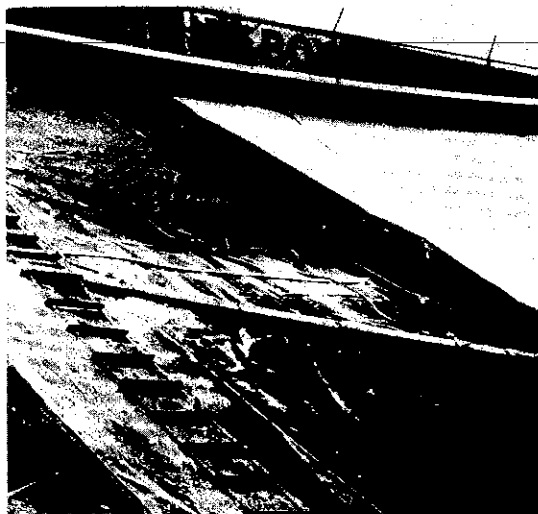
Figure A-20. Support board for working on steep incline.
