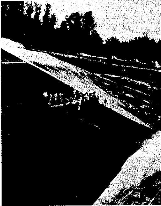
Figure A-24. Field seams parallel to side slope toe.
