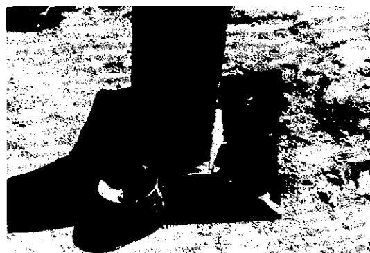
Figure A-39. Liner pad around a concrete penetration.
