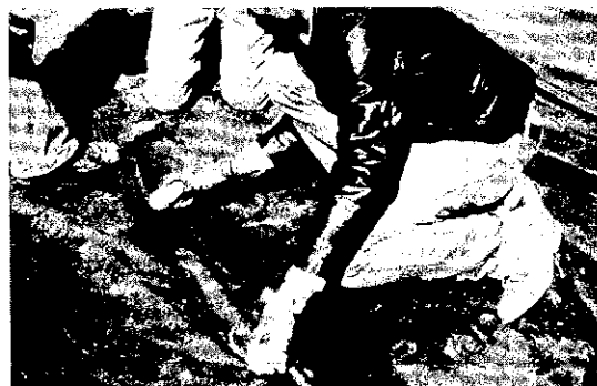
Figure A-21. Unsuccessful seaming with a solvent adhesive in cold temperatures.
