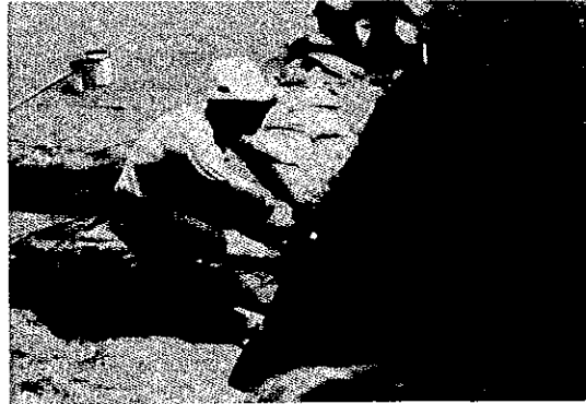
Figure A-26. Plastic dowels being used to pull liner panels.
