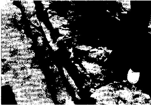
Figure A-13. Initial placement of a liner into an anchor trench.
