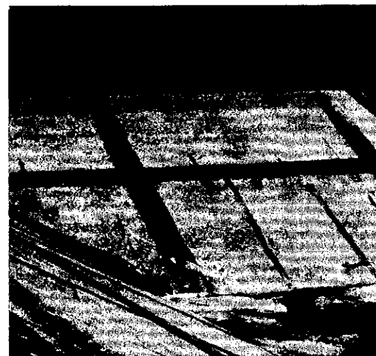
Figure A-23. Patching compounds applied to concrete panel joints.
