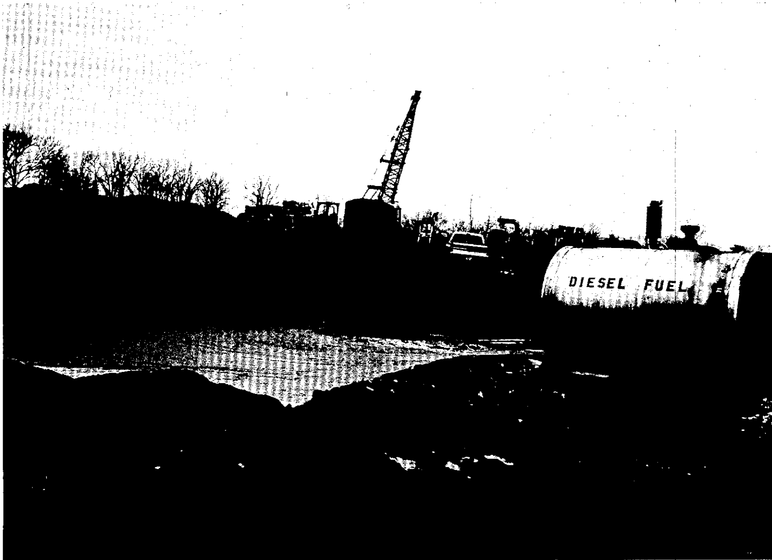
Figure 6-10. Removal of Ash Deposits Near Slurry Discharge, Gibson Station
