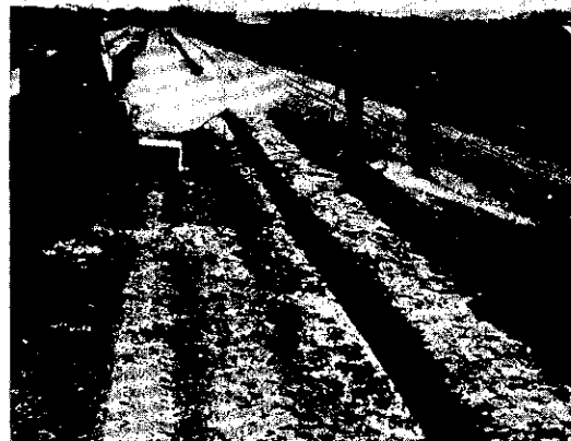
Figure A-11. Application of an herbicide to the subgrade for soil sterilization.
