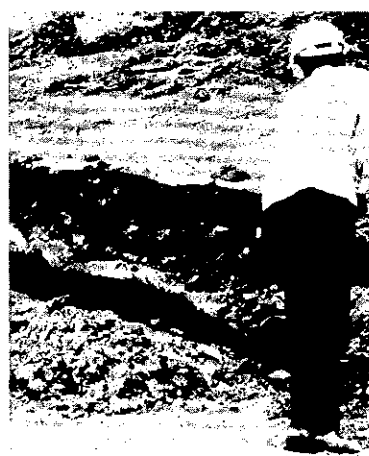
Figure A-64. Exposing edge of liner for expansion.
