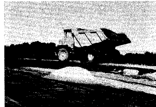
Figure A-52. Large dump truck placing soil cover.
