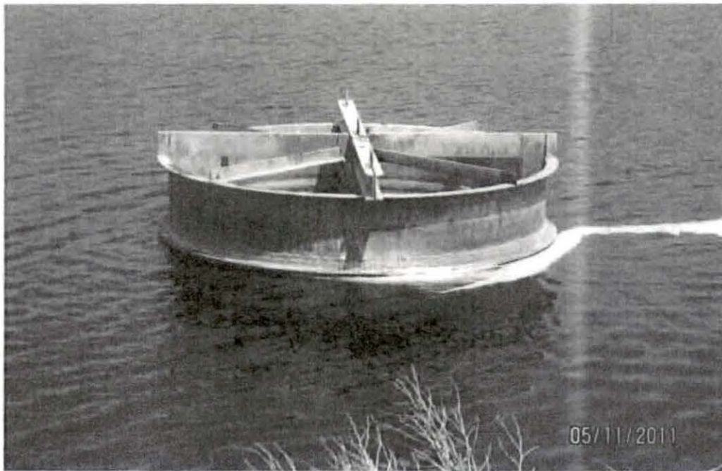
Photograph 7. Riser in CAPE FEAR 1985 coal ash basin from 2012 Five Year Independent Consultant Report.
