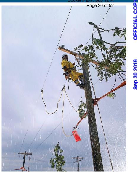
**LINEMAN IN RAIN** IN AREAS INACCESSIBLE BY BUCKET TRUCK, LINEMEN HAVE TO CLIMB POLES TO MAKE REPAIR same reliability benefits as a modern transformer installed today.
