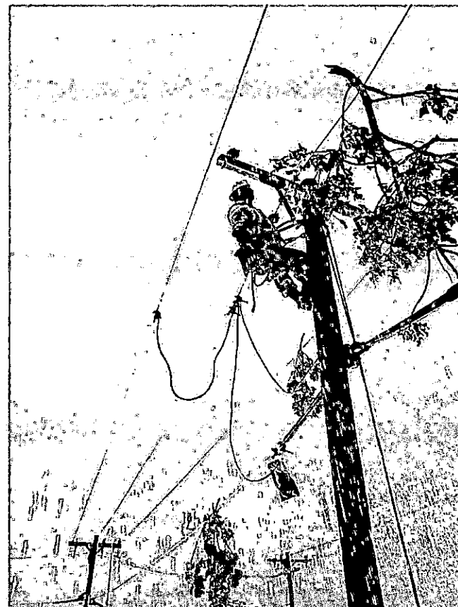
LINEMAN IN RAIN IN AREAS INACCESSIBLE BY BUCKET TRUCK, LINEMEN HAVE TO CLIMB POLES TO MAKE REPAIR
