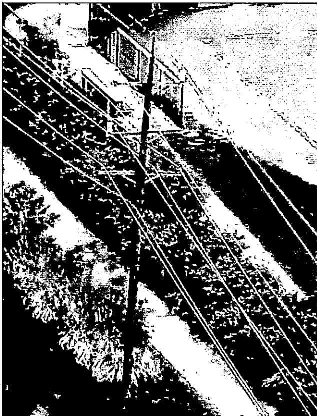
69 KV WOOD POLE CONSTRUCTION
