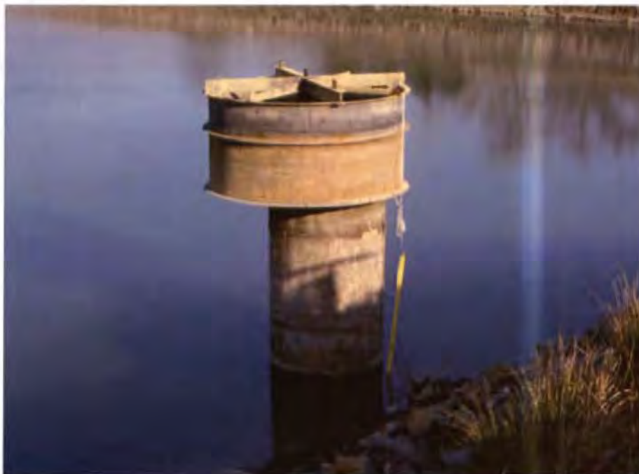
Photograph 12. 3/19/14 photograph of CAPE FEAR 1985 coal ash basin riser, prior to repair work.
