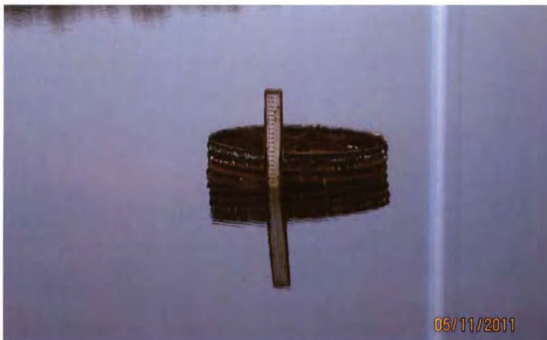
Photograph 6. Riser in CAPE FEAR 1978 coal ash basin from 2012 Five Year Independent Consultant Report.
