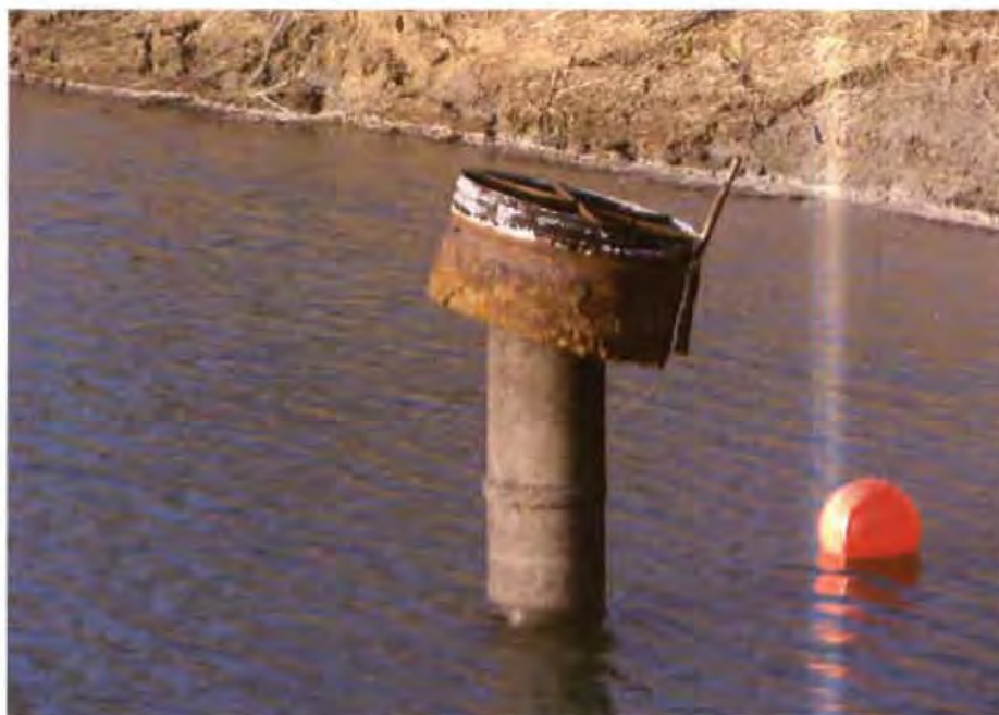
Photograph 11. 3/19/14 photograph of CAPE FEAR 1978 coal ash basin riser, prior to repair work.
