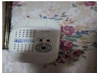
Non-Functioning CO Detector
