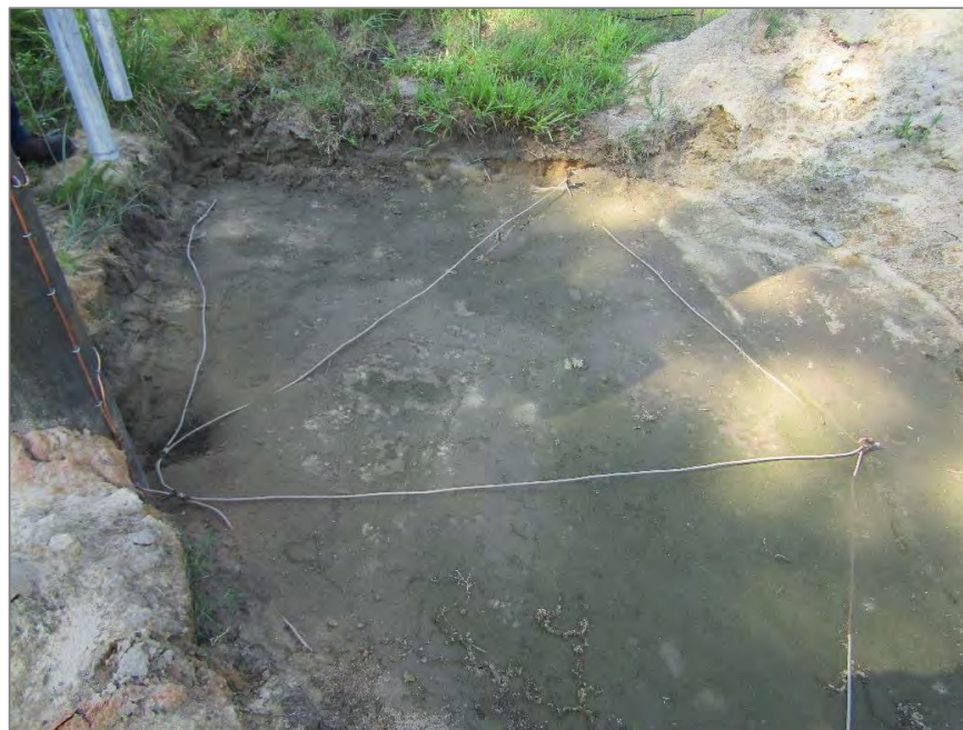
Duke Energy GOAB ground grid with 2 AWG bare solid copper wire grid loop and four ground rods
