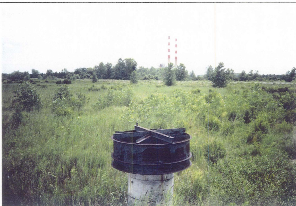
PHOTO #8 - Photo of the overflow pipe to the old fly-ash pond at the southwest corner of the site. Approximate location of GW02.
